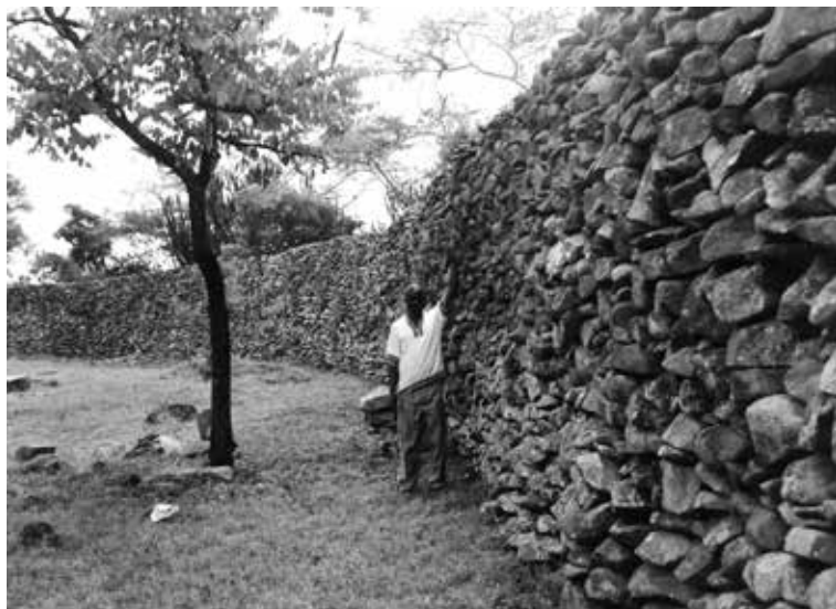
Enclosure wall with buttress. External walls range in height from 0.5–4.2m, with a thickness of 1m. They were made of loose stone without any dressing or mortar, and care must have been taken to ensure their stability.
