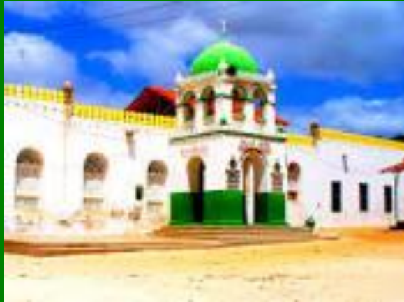
The Riyadhha Mosque in Lamu: Kenya's latest National Monument (see p. 10)
